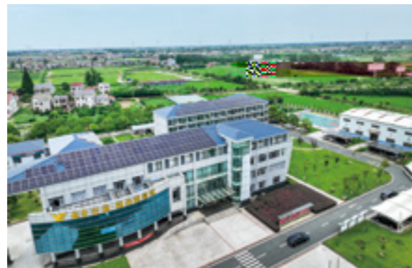
Yuexiu Transport Suizhou-Yueyang Expressway South Section PV project
